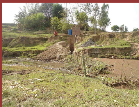
Newly installed water-pump, BASE, West Nepal
